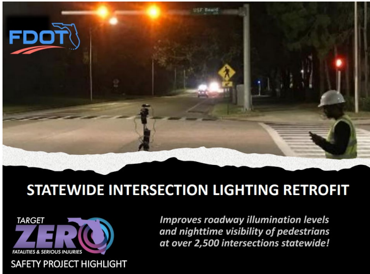
Retrofitting pedestrian lighting at signalized intersections
